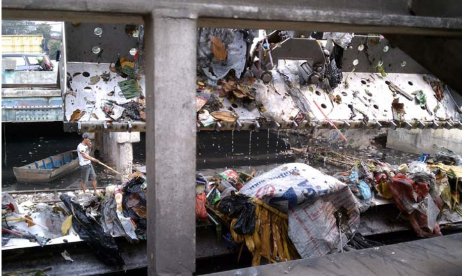
Pneumatic rake of a trash gate transferring refuse onto a conveyor belt
