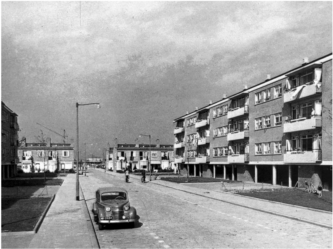
Street in Pendrecht, Rotterdam.
