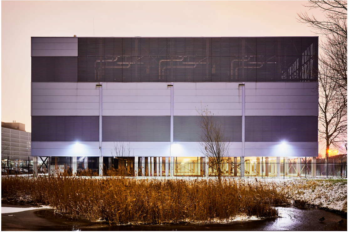
Equinix AM5 Datacenter, Amsterdam.
