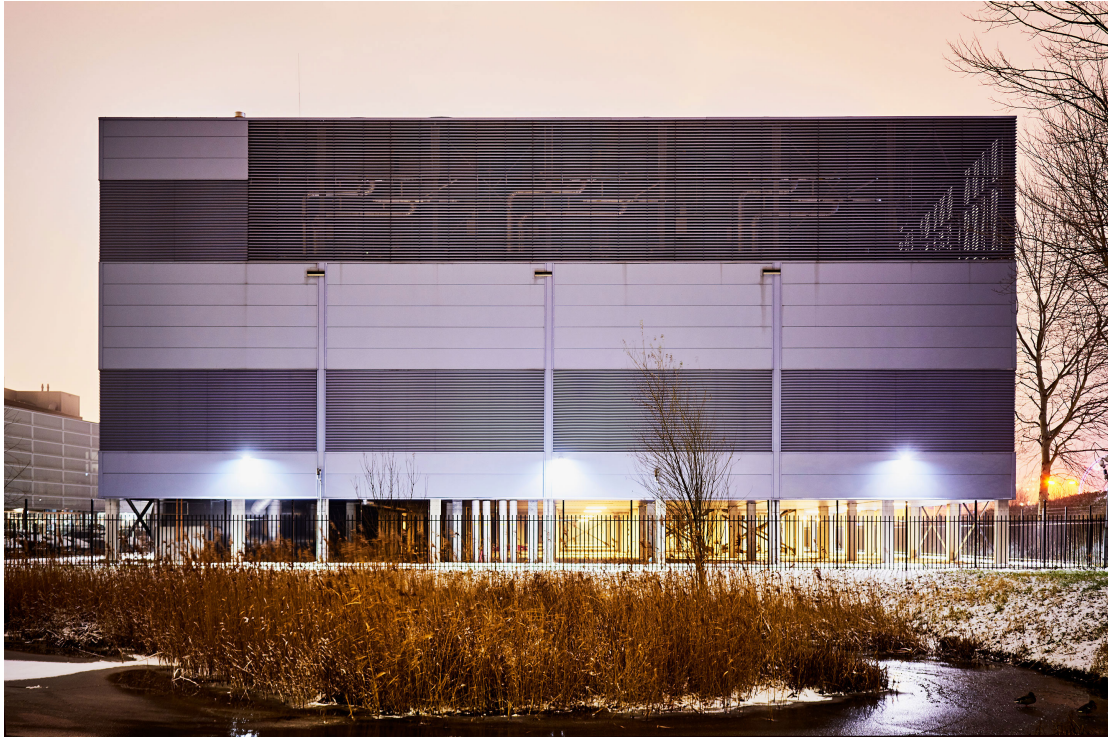
Equinix AM5 Datacenter, Amsterdam.
