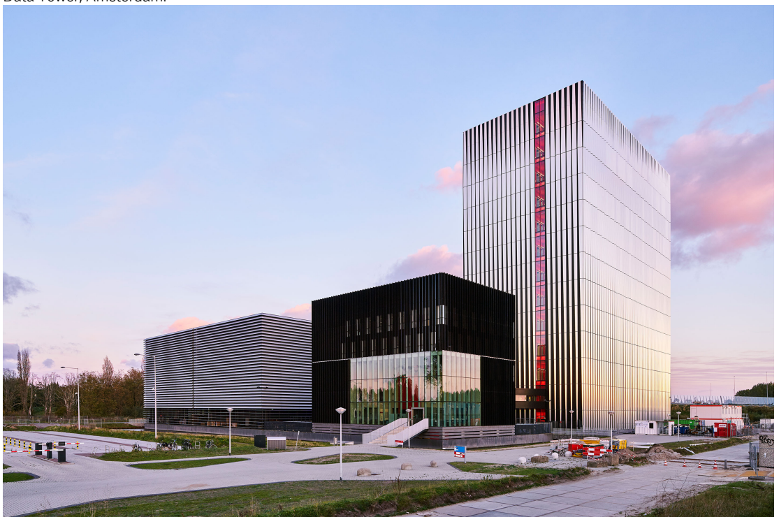
Equinix AM4 Datacenter, Amsterdam.
