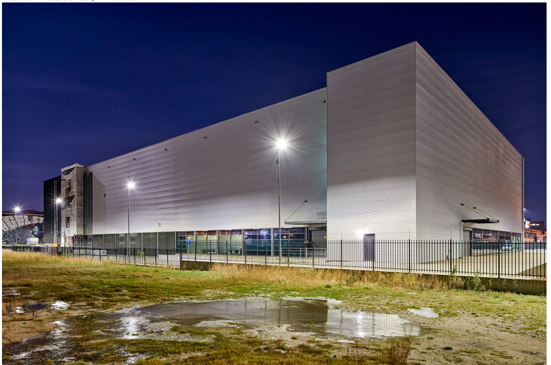
Equinix AM6 Datacenter, Amsterdam.
